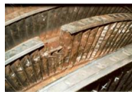
Figure 5. The example of destruction or damage of the turbine blades
